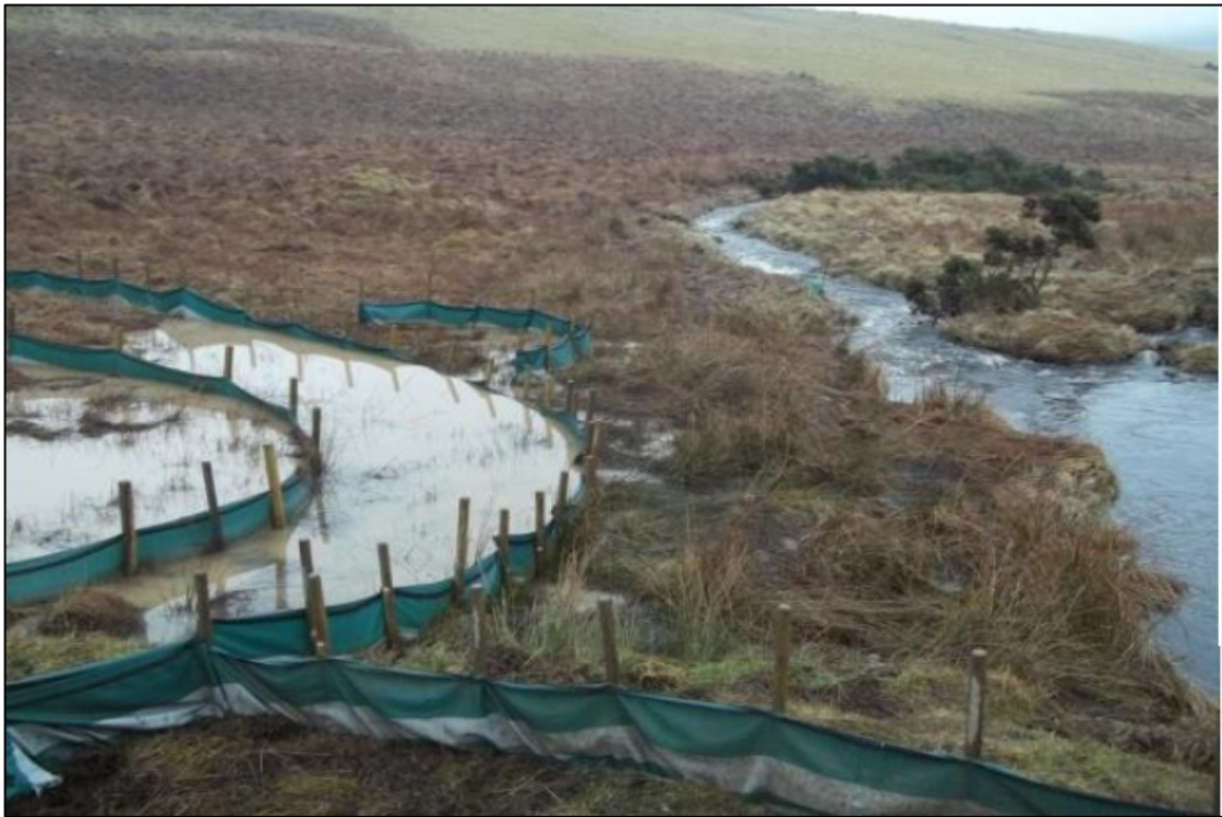
Plate 5.2: Photograph of Silt Fencing
