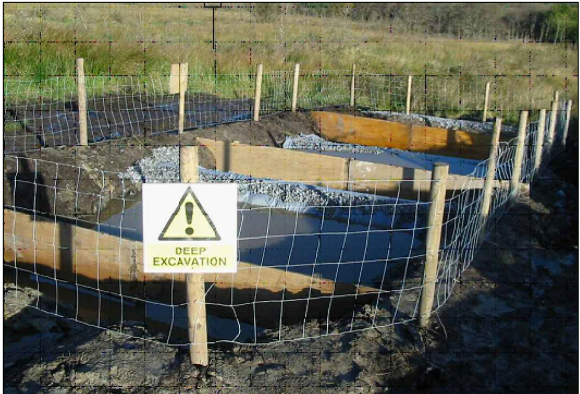
Plate 5.4a: Completed Settlement Pond System
